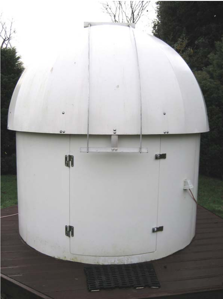
Figure 5.1. Illustrating how the dome aperture guiding rails can block the opening and closing of the door on the Pulsar Optical 7-foot dome. In this photograph I have the door facing north, and the aperture facing south where most of my imaging takes place.
