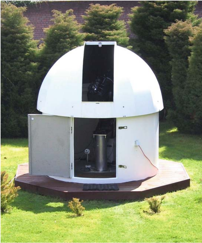
Figure 1.7. The Pulsar Optical 7 foot diameter fibreglass dome in its back-garden location in the New Forest, Hampshire, U.K. The dome sits on a hexagonal 10-foot diameter wooden decking.
